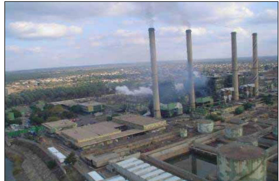
Doura Thermal Power Plant, Baghdad
