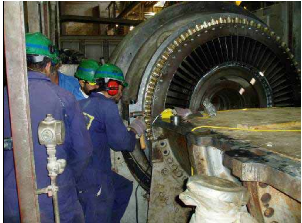
Iraqi Engineers rebuild a GE Frame 5 (22MW) Gas Turbine near Basra.
