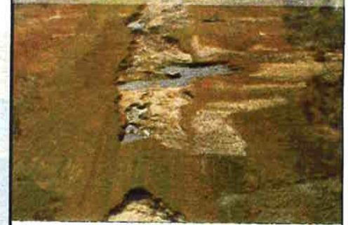
Btw control structures - MRGO
