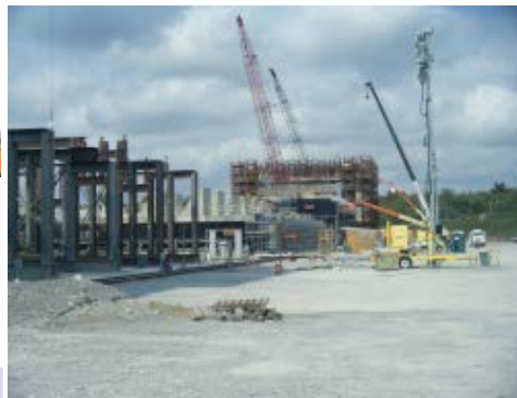
Above: Land Construction Site
