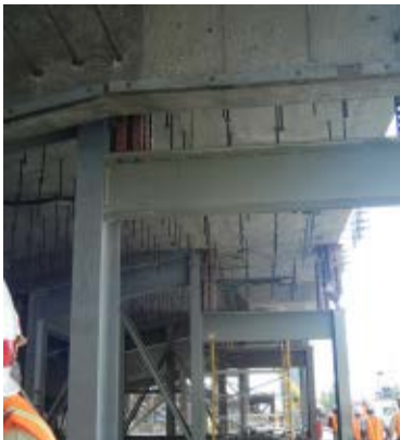
Above: Underneath Stilling Basin Shell
